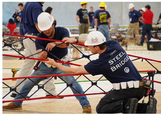
LU team members connect beams of the bridge during the competition hosted by Louisiana Tech over the weekend. (Photo by Logan Grasser)
