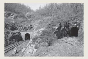
The 4,273-foot Crozet's Blue Ridge Tunnel was the longest railroad tunnel in North America when constructed in 1849–1858. Irish and enslaved craftsmen and laborers excavated the tunnel using hand drills and black powder. Chief Engineer Claudius Crozet designed a singular elliptical cross-section to minimize rock removal. Its slope from west to east presented challenges for drainage and ventilation. Crozet developed unique solutions to these problems. In April 1858, the first train
