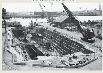
The War of 1812 taught America the importance of a strong navy. Designed by Loammi Baldwin, Jr. and completed in 1834, Dry Dock No. 1 at the Norfolk Naval Shipyard was of a size and complexity not previously known in the United States. Measuring 314 feet long and 100 feet wide, the dry dock was constructed with New England granite and utilized eight lift pumps powered by steam engines. This dry dock, as well as its companion dry dock in the Boston Navy Yard, strength-
