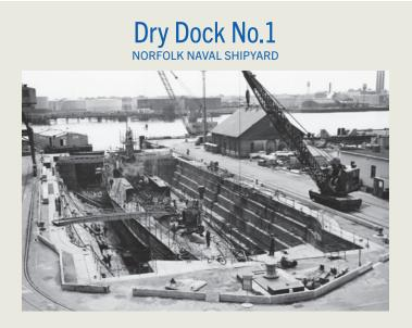
The War of 1812 taught America the importance of a strong navy. Designed by Loammi Baldwin, Jr. and completed in 1834, Dry Dock No. 1 at the Norfolk Naval Shipyard was of a size and complexity not previously known in the United States. Measuring 314 feet long and 100 feet wide, the dry dock was constructed with New England granite and utilized eight lift pumps powered by steam engines. This dry dock, as well as its companion dry dock in the Boston Navy Yard, strength-
