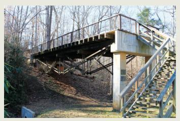
This 56-foot, single-span Fink deck truss was built around 1870 to carry trains of the Atlantic, Mississippi and Ohio Railroad (now the Norfolk Southern Railway). The original location of this structure is unknown. In 1893 it was relocated to carry Old Forest Road over the Norfolk and Western Railway in Lynchburg, Virginia. In 1985 the bridge was again relocated to Riverside Park in the City of Lynchburg to preserve its historic significance. This structure is notable
