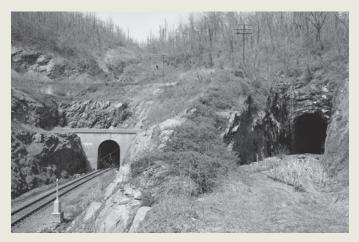
The 4,273-foot Crozet's Blue Ridge Tunnel was the longest railroad tunnel in North America when constructed in 1849–1858. Irish and enslaved craftsmen and laborers excavated the tunnel using hand drills and black powder. Chief Engineer Claudius Crozet designed a singular elliptical cross-section to minimize rock removal. Its slope from west to east presented challenges for drainage and ventilation. Crozet developed unique solutions to these problems. In April 1858, the
