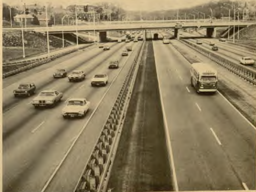
Urban expressways increasingly became arteries for public mass transportation in the early 1970s, as illustrated by these reserved bus lanes on the Shirley Highway.
