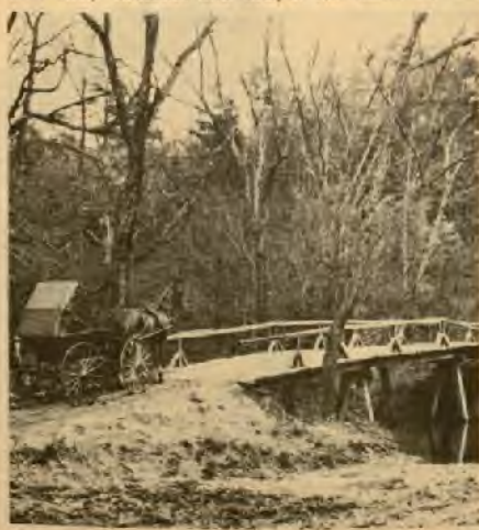
This bridge, constructed in the 1870s, was typical of many in rural Virginia at the turn of the century.
