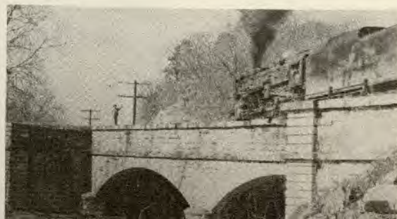
C & O Railway Crossing a James River Canal Aqueduct, near Hardware, Virginia—Preston Leech.
