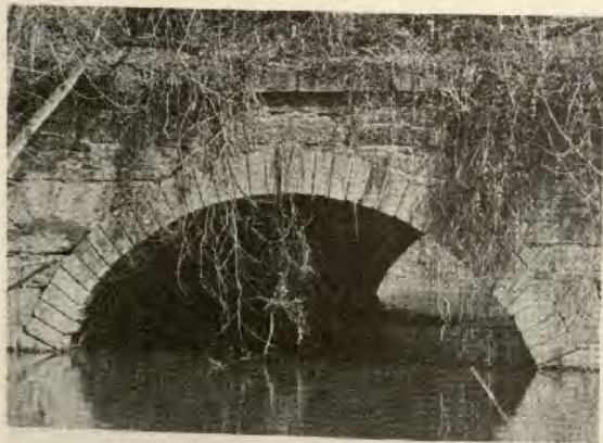
Viaduct Crossing (location known)—Preston Leech.
