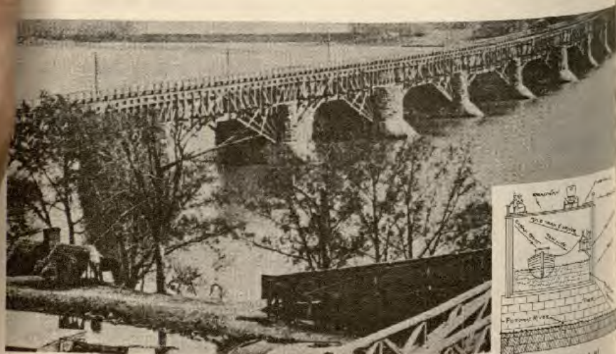
For 30 years this aqueduct served canal boats, carriages, and pedestrians crossing the Potomac at Georgetown. Inset: A diagram of the aqueduct.
