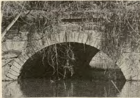
Viaduct Crossing (location known)—Preston Leech.
