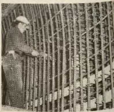
Reinforcing of tunnel lining—VDH.
