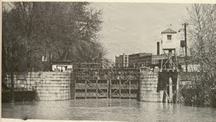
The Ship Lock, Tidewater Connection, at Richmond, Va.—Preston Leech.
