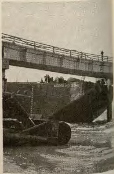
Barge Being Removed from Bridge After the Storm of October 1972 (Courtesy Virginia Dept.
