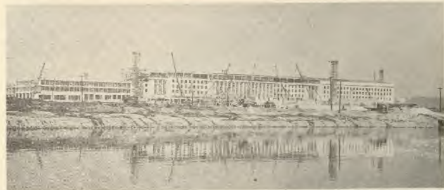
SC 647320 Construction of the River Entrance to the Pentagon.
