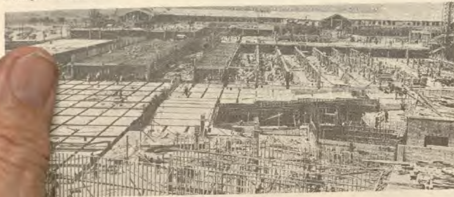
318 Construction of the —Forming of Floors.
