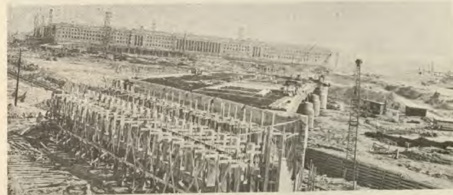
SC 647822 Construction of the Pentagon—Ramp and Overpass.
