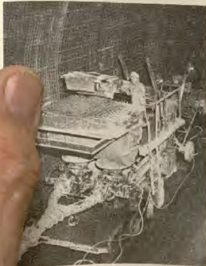
Concrete placing equipment—
