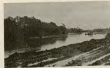
SC 647809 Construction of the Pentagon—Flooding of Excavation.
