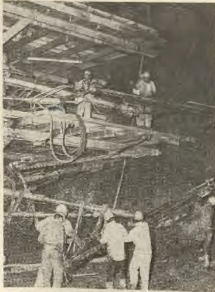
Platform and Drills for Rock Excavation in the Tunnel—VDH.
