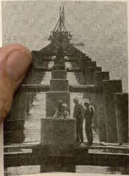
Trestle Piling in Place Ready for
