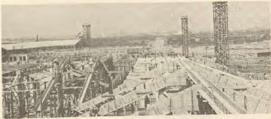
SC 647316 Construction of the Pentagon—Forming.
