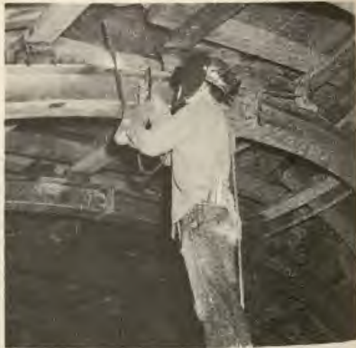
Welding Structural Ribs for the Roof of the Tunnel—VDH.
